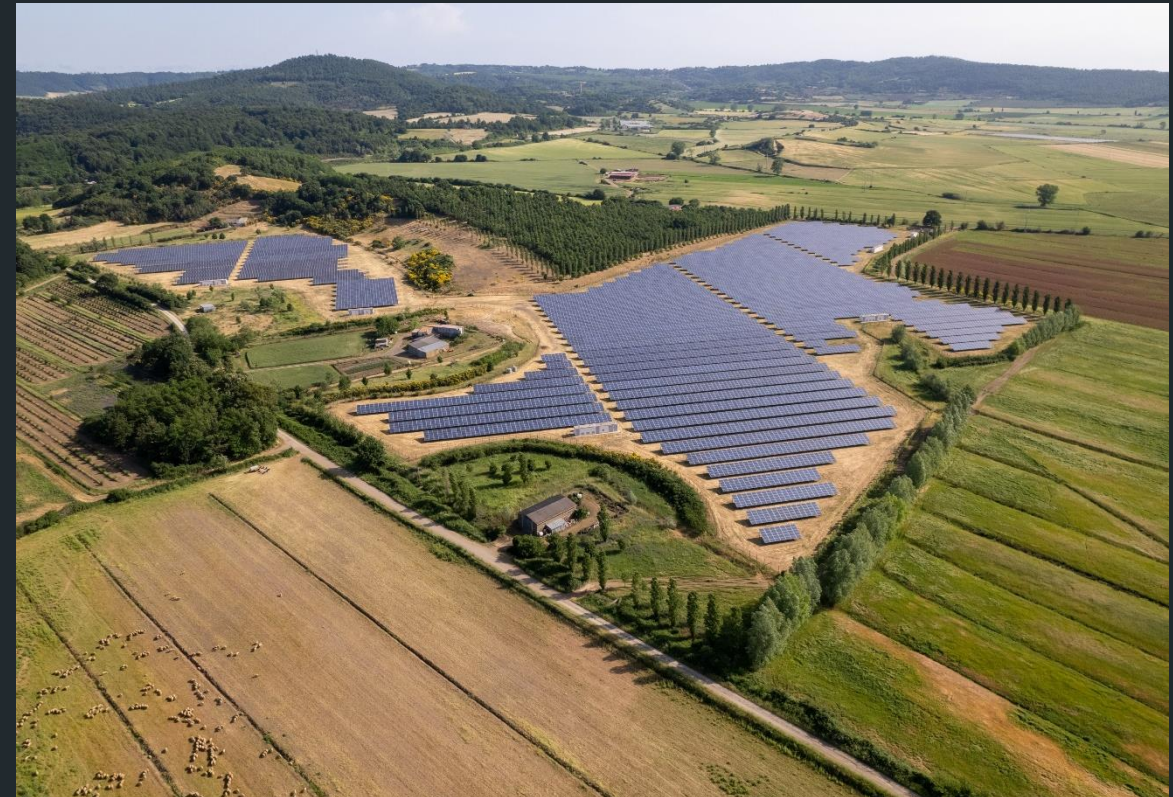
Solar PV Plant
